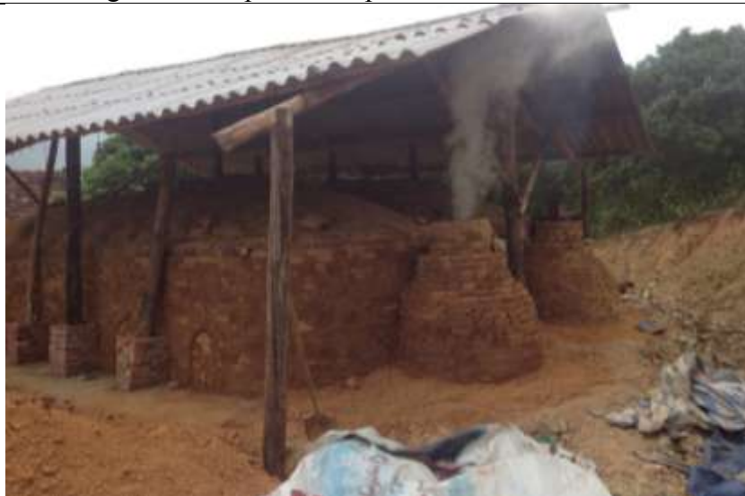
Check Smoke to prepare next step
